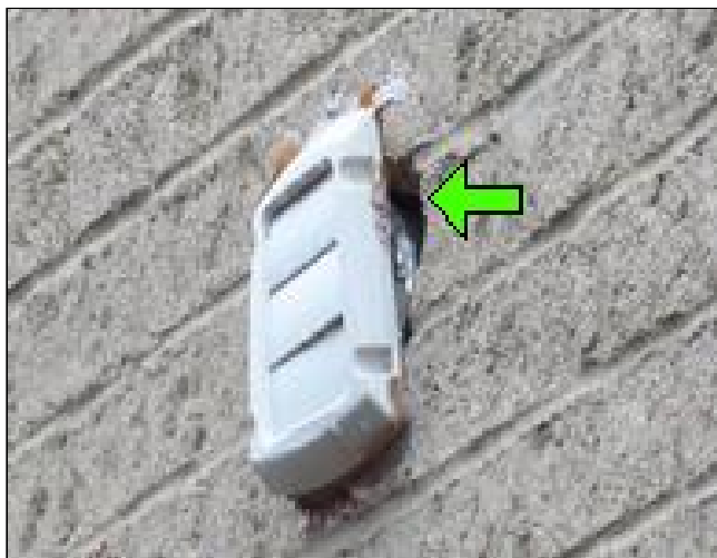
7.4 Item 4(Picture) If the duct is not metal upgrade it.
