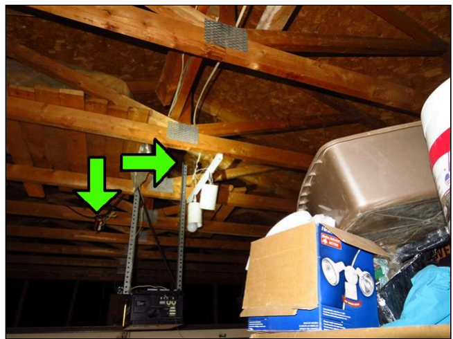
8.3 Item 2(Picture) Open splices. Loose wires.
