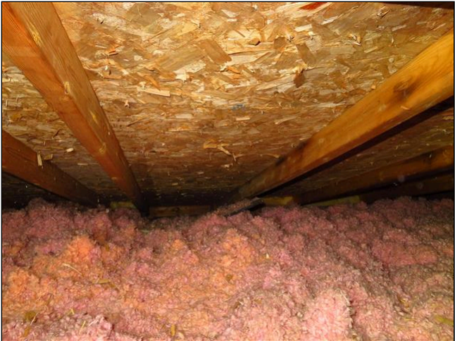
7.0 Item 2(Picture) Compressed (damaged) material
